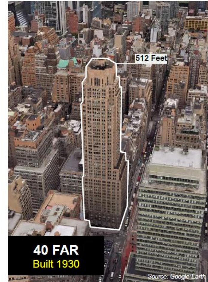
The Navarre Building in the Northwest Plan Area
